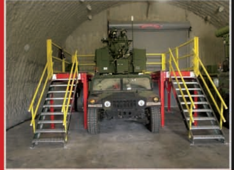
FORT BRAGG HUMMER ACCESS MEZZANINE
